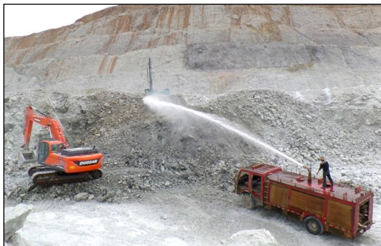
Figure 18-1: On-site Water Sprinkling
