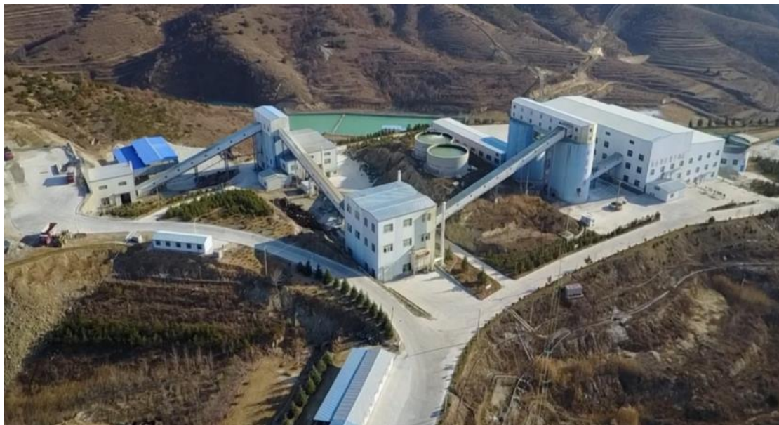
Figure 15-2: Aerial Photo of the Processing Plant
