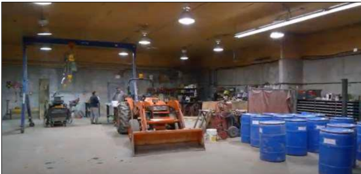
Figure 18-3: Existing Surface Shop
