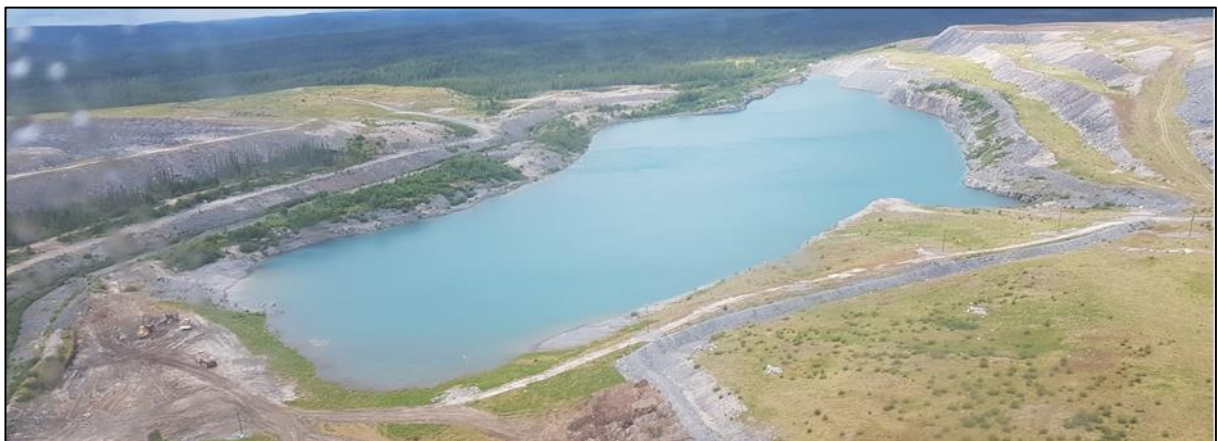
Figure 4-7: Troilus J Zone Open Pit (looking northwest)
