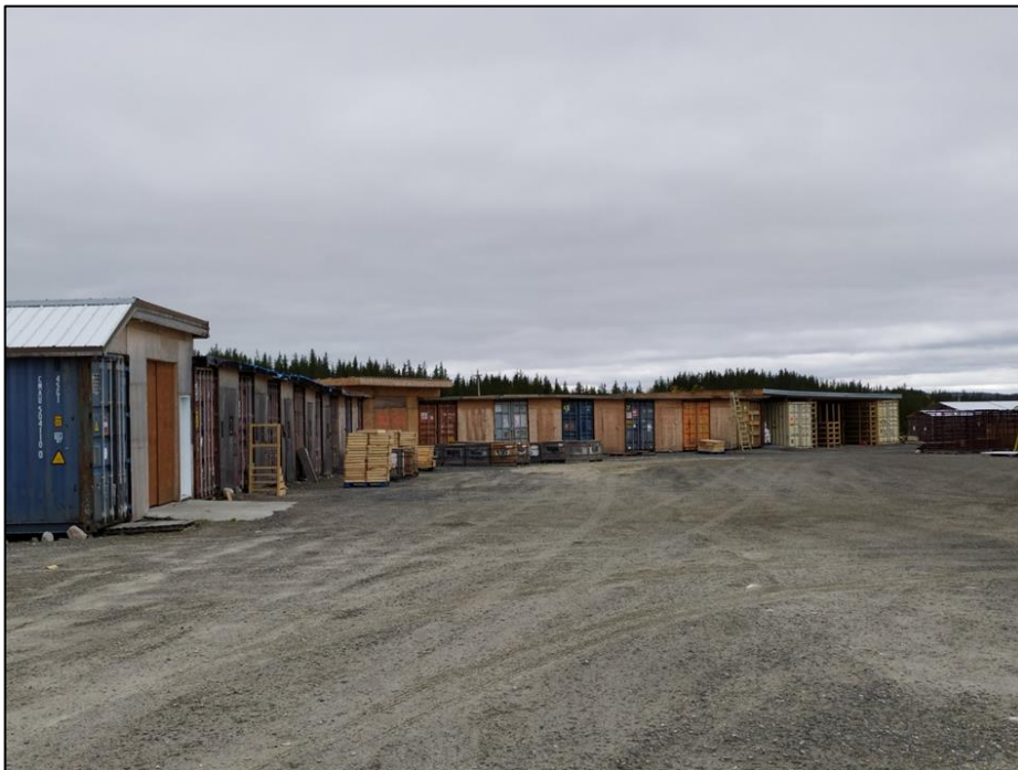
Figure 12-5: Core Storage Area; Pulp and Rejects Storage Facility
