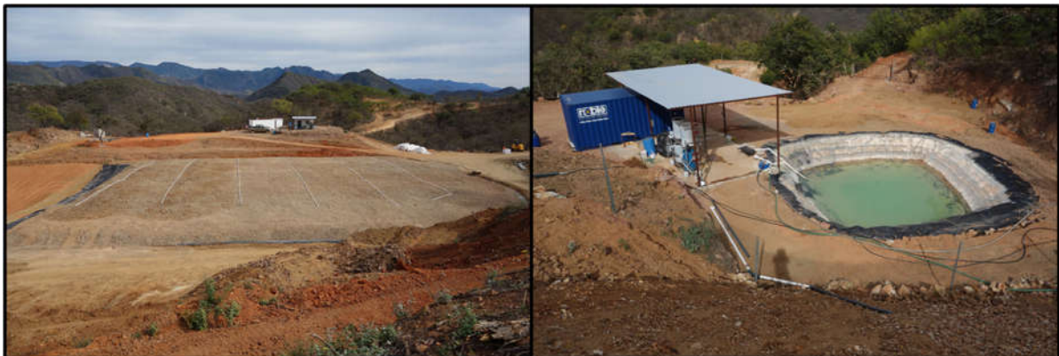
Figure 4-3: Bulk Heap Leach Pad and Test Plant
