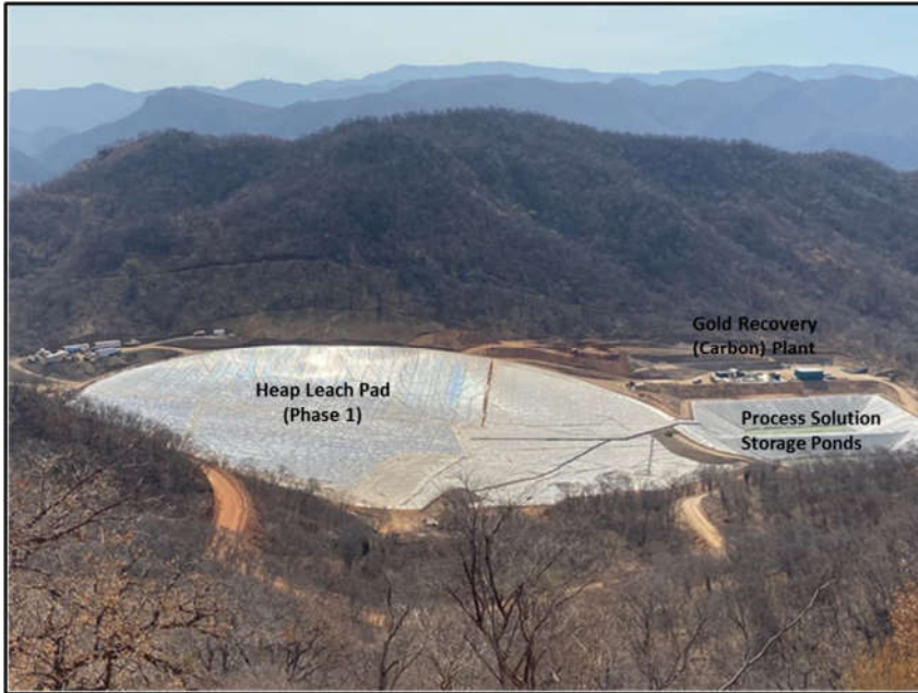
Figure 18-3: Heap Leach Pad and Process Storage Ponds
