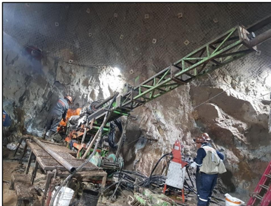
Figure 10.3 Drill Bay at Huayra Kasa Adit
