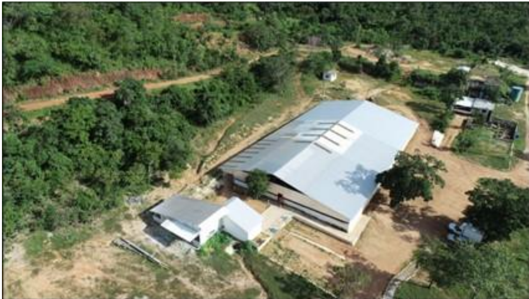
Figure 5.3 – Cerrado Gold Core Logging Area and Office
