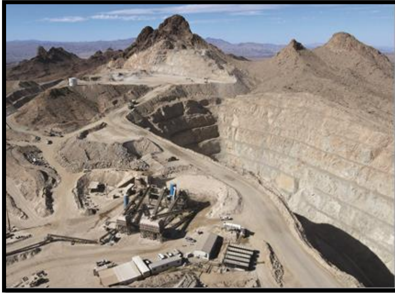
Figure 23.1-1 Moss Mine Pit (E&MJ 2022)
