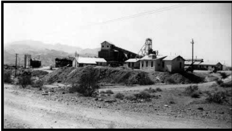
Figure 14.4-1 The headframe and mill buildings at the Katherine mine, circa 1930s, ADMMR Photo Archive, Arizona Geological Survey.
