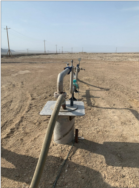
Figure 13-2: Brine Extraction Well at Silver Peak
