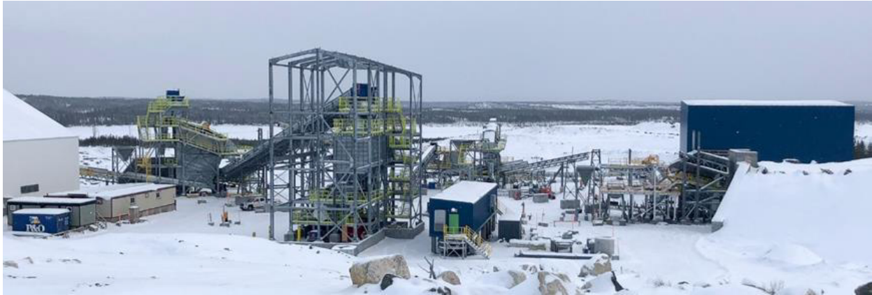
Figure 24-1 View of Primary and Cone Crusher Buildings
