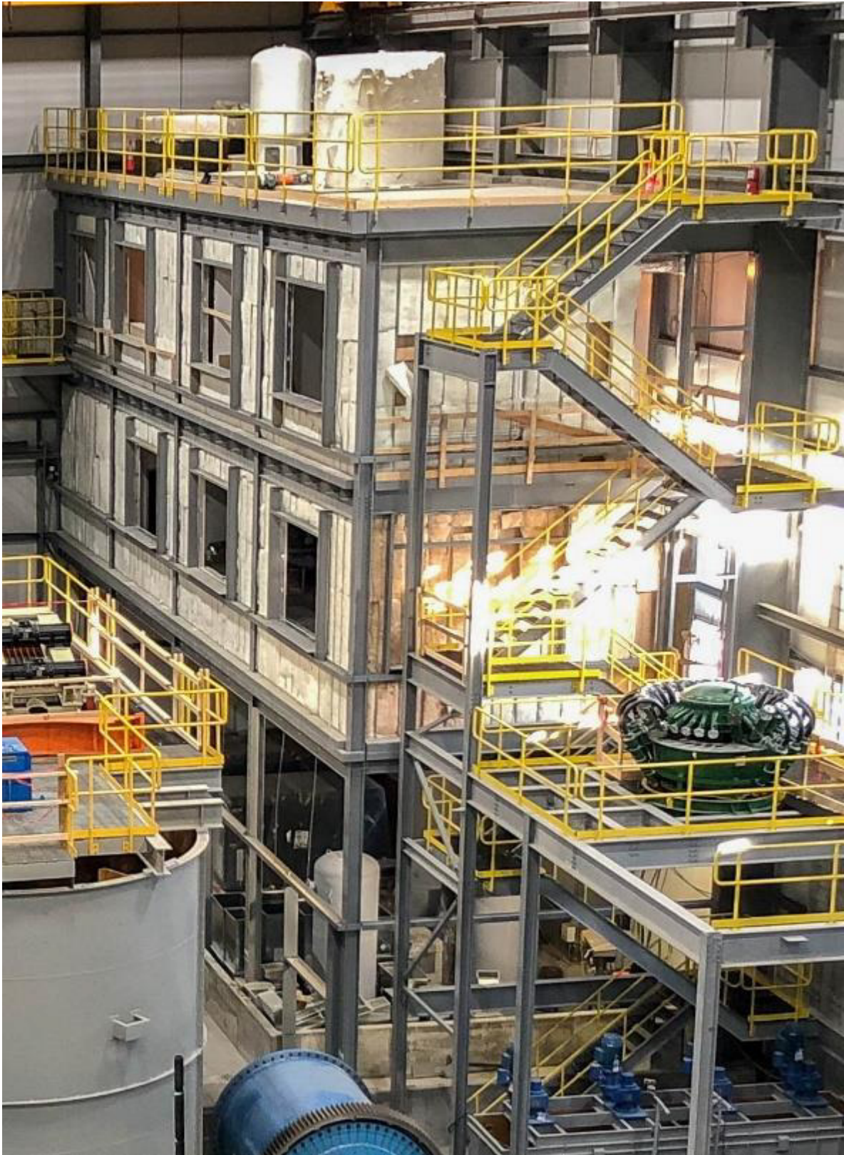
Figure 24-4 View of Offices and Control Room
