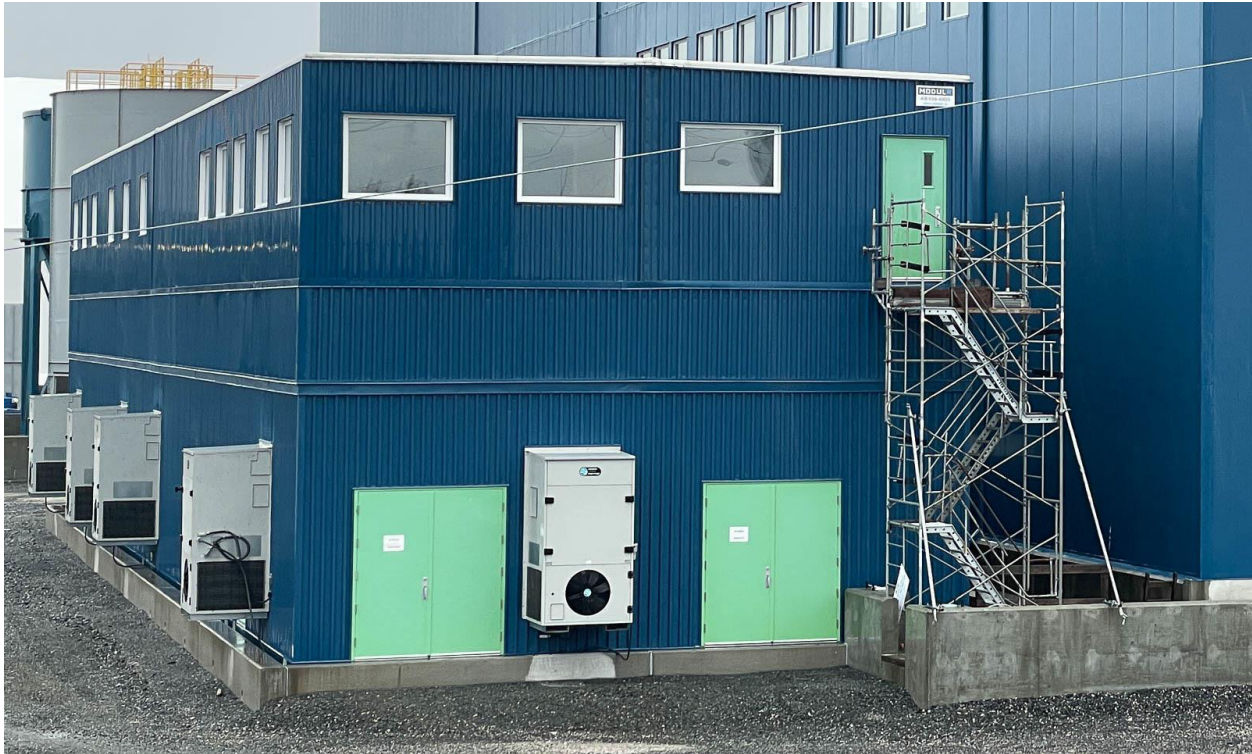
Figure 24-11 Concentrator Main Electrical Room, Offices and Laboratory
