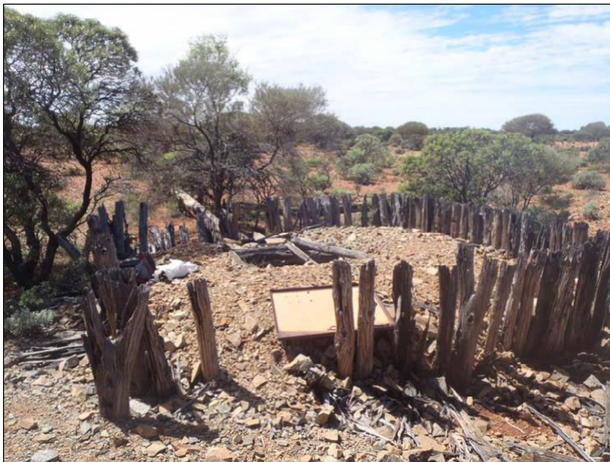
Figure 37 The mining shaft at the Homeward Bound prospect now reused as a water point by pastoralists.
