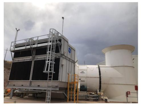
Figure 18.4: Air Intake through Cooling Fins with Cooled Air Delivered to the Underground
