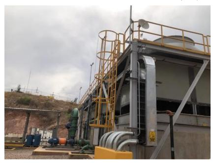
Figure 18.3: Evaporative Cooling Towers as the First Stage of Cooling
