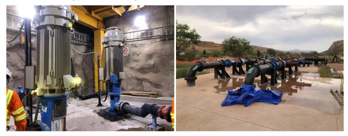
Figure 18.5: Underground Wellhead Pumps and Surface Discharge Header
