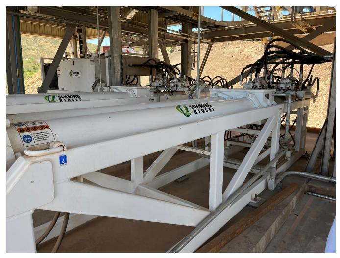
Figure 18.10: Positive Displacement Pumps for Paste Fill
