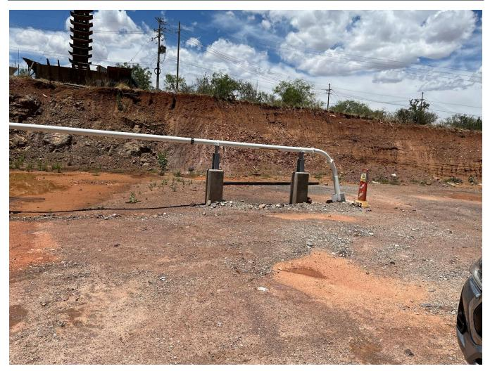
Figure 18.11:Paste Surface Pipeline to Borehole
