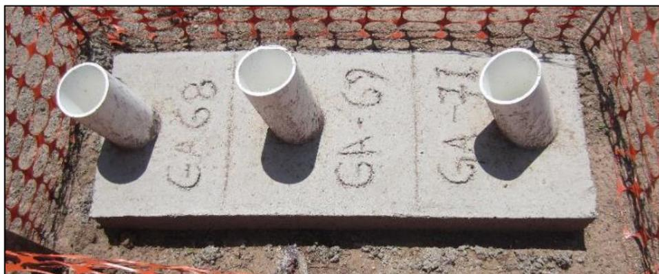
**Figure 10.5: Example of a Completed Drill Hole Site****10.1.3.3.2 Underground Drill Holes**
