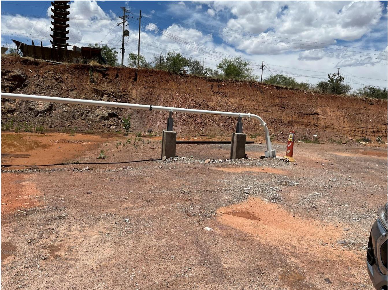
Figure 18.11: Paste Surface Pipeline to Borehole
