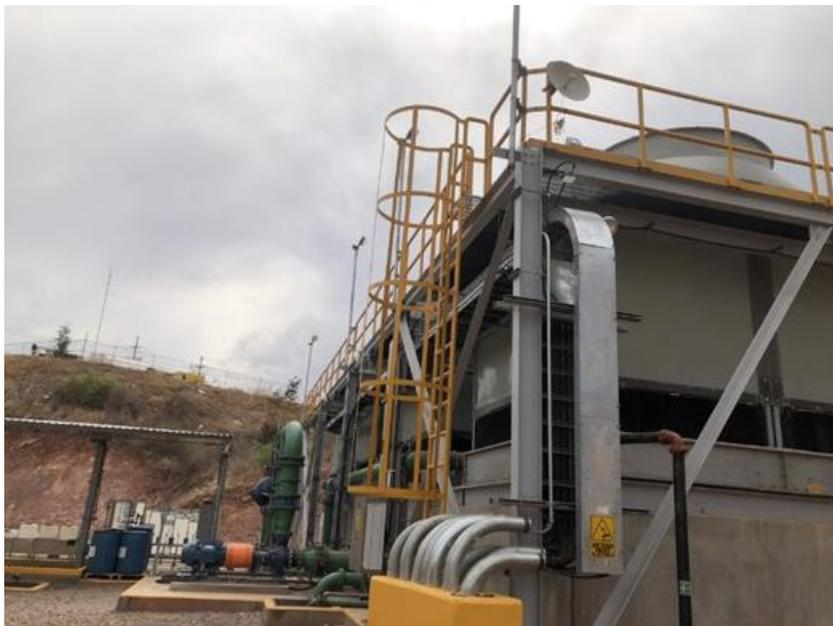
**Figure 18.3: Evaporative Cooling Towers as the First Stage of Cooling**
