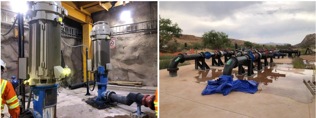
Figure 18.5: Underground Wellhead Pumps and Surface Discharge Header
