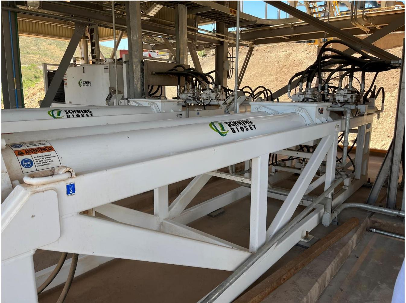
Figure 18.10: Positive Displacement Pumps for Paste Fill
