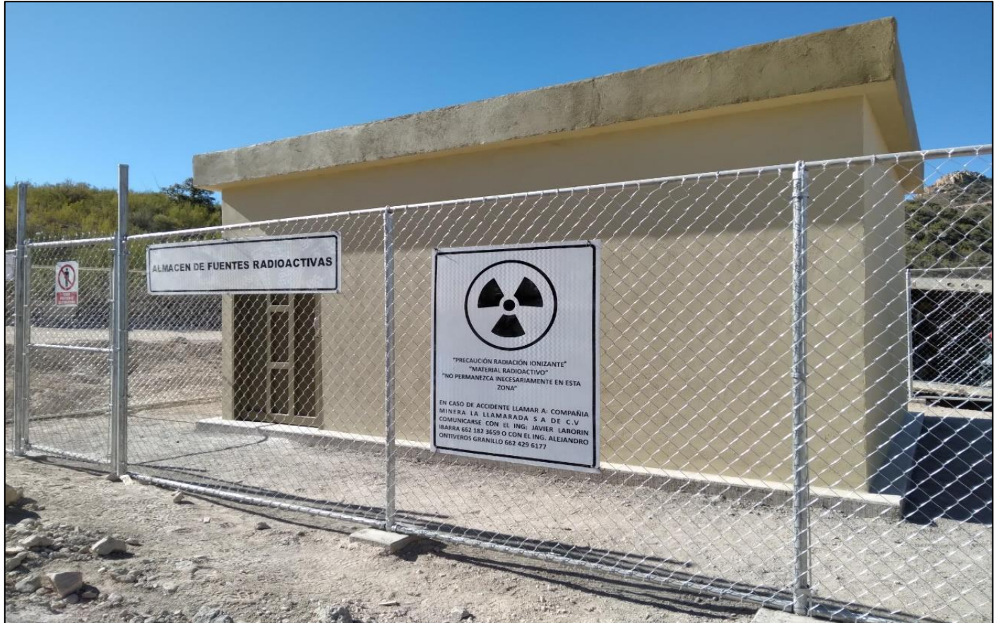
Figure 18-19: Nuclear Devices Storage Facility
