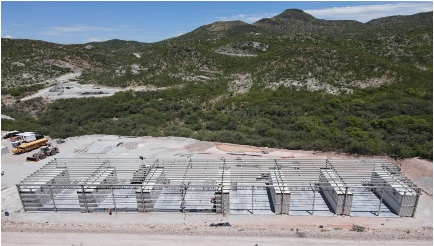
Figure 16-32: Surface Maintenance Shop – Construction View
