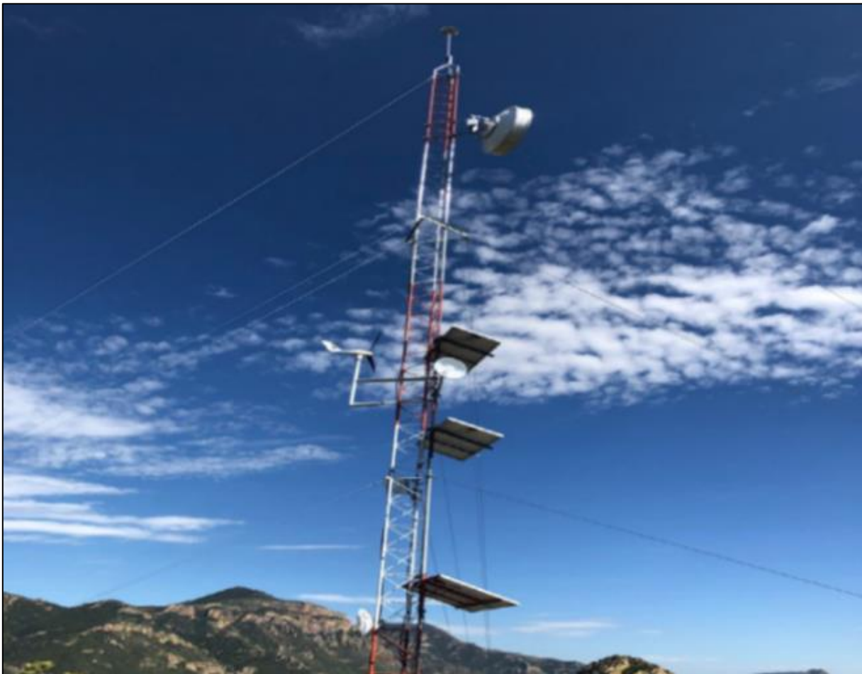
Figure 18-13: Communication Tower located at Babicanora Hill
