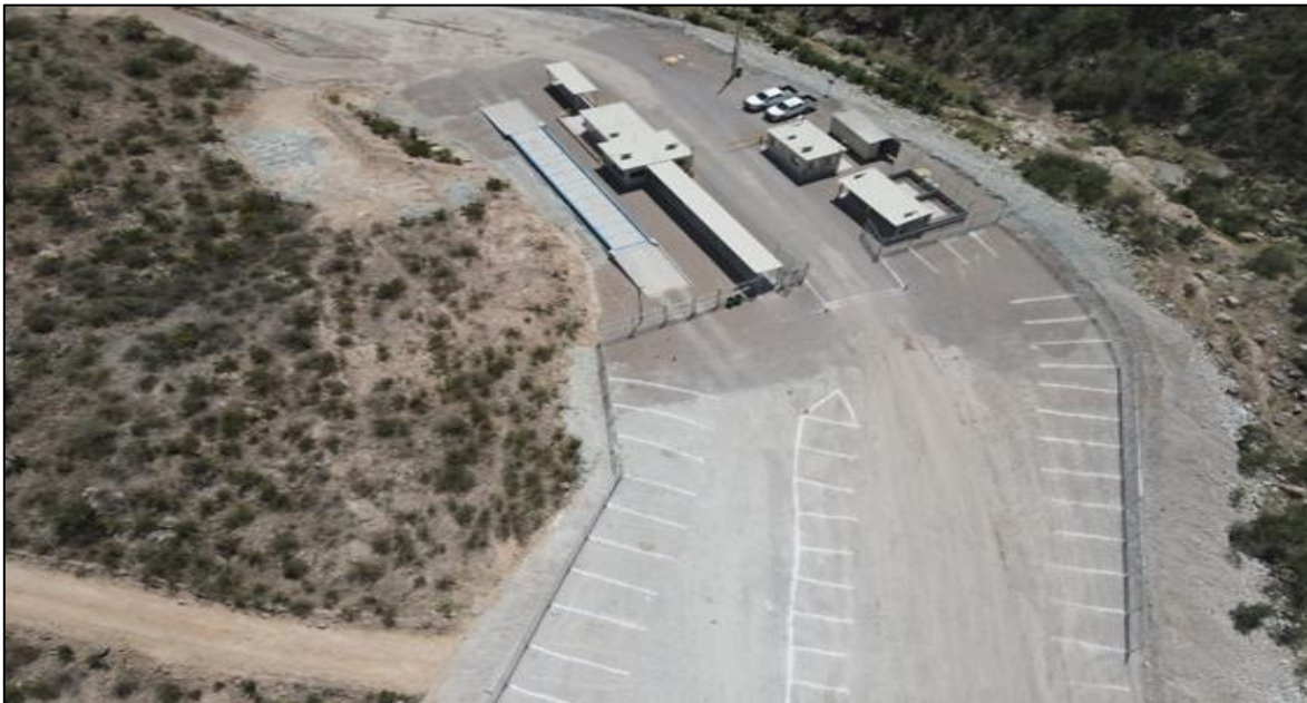
Figure 18-5: Security Gate #2 (Main access point)
