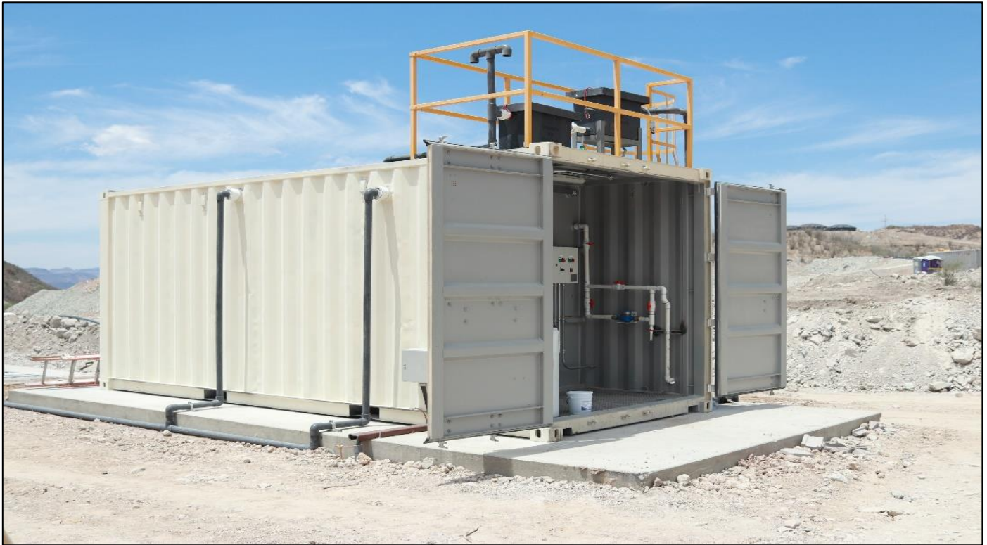
Figure 18-16: Sewage Treatment Module
