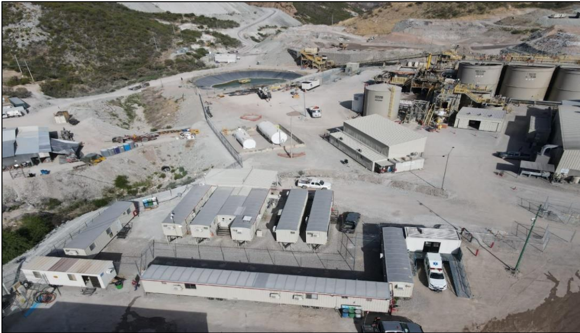
Figure 18-25: Process Plant Office
