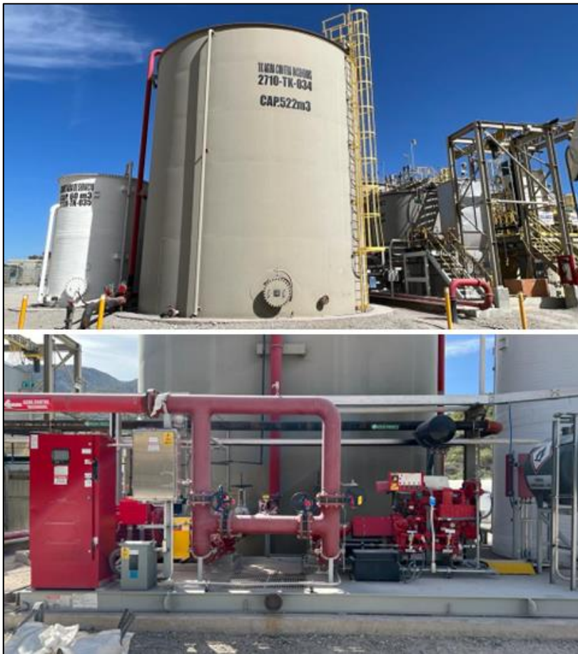
Figure 18-14: Fire Water Supply and Distribution Systems
