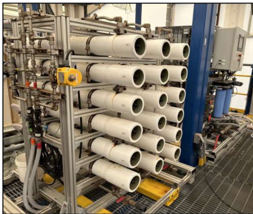
Figure 13-6. Osmotically Assisted Reverse Osmosis System at the Demonstration Plant
