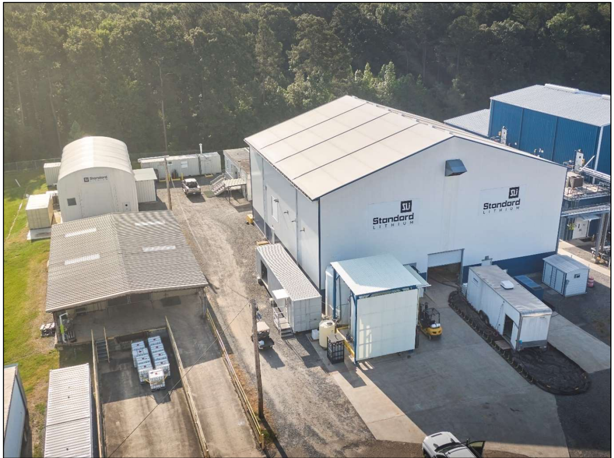
Figure 13-2. Standard Lithium Demonstration Plant
