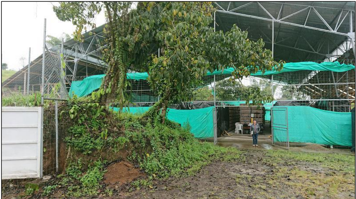
Figure 11-1: Core Shed at the Chorroseco Site with Metal Fences and Security for Old Core Storage
