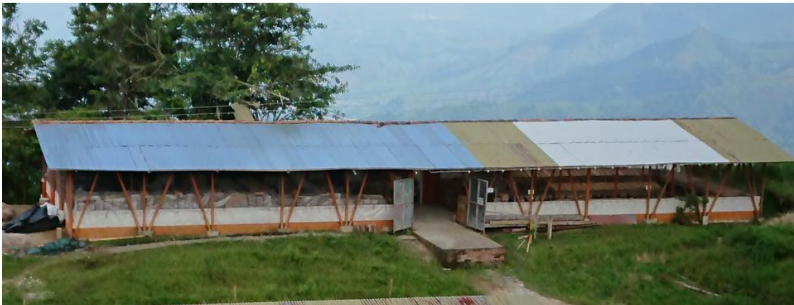
Figure 10-5: Core Warehouse and Logging Facility at La Cumbre Site
