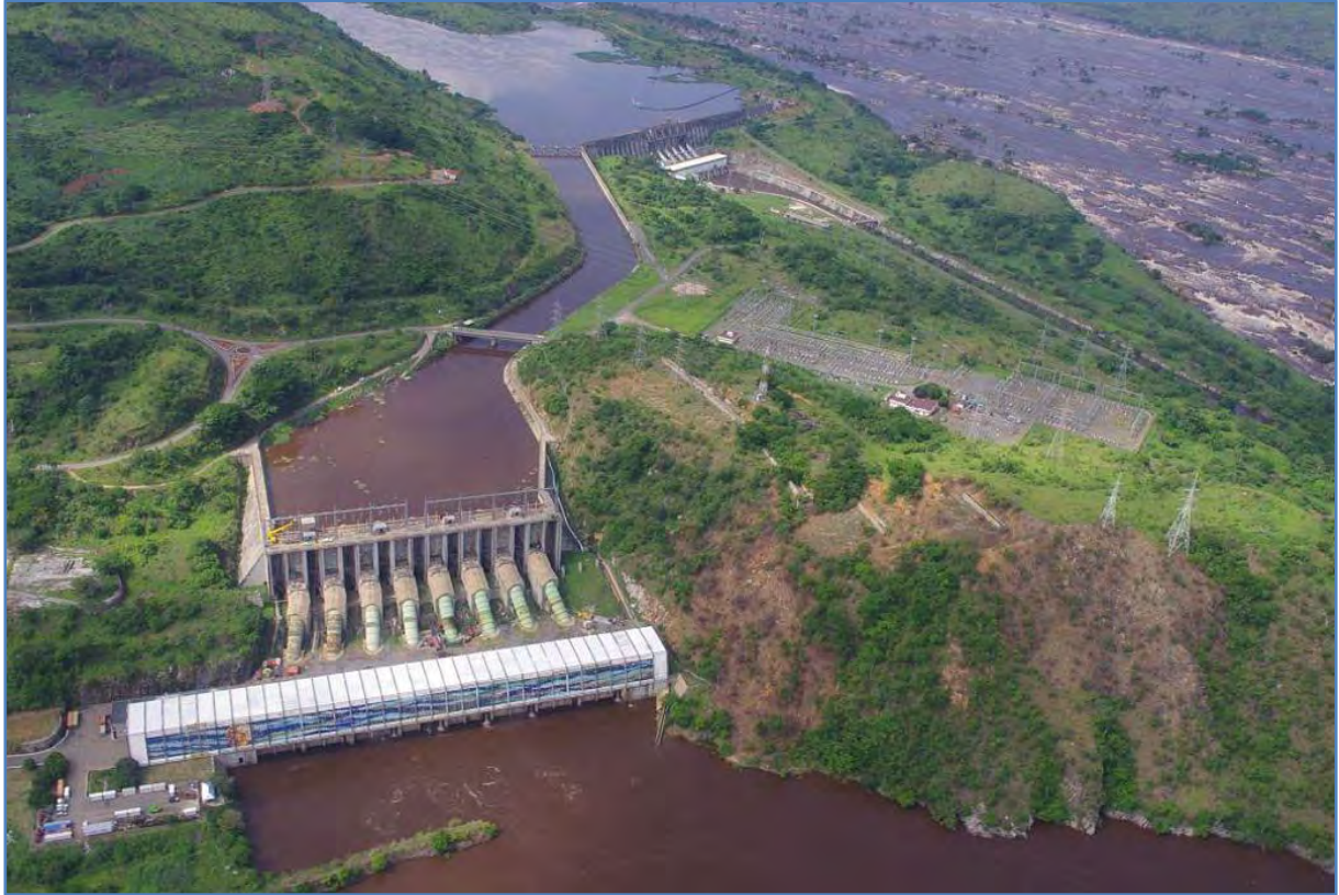
Figure 18.5 Inga II Hydropower Plant
