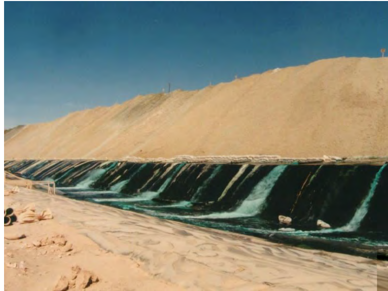
Figure 14-12: Ore on pad with solution flowing to toe drain
