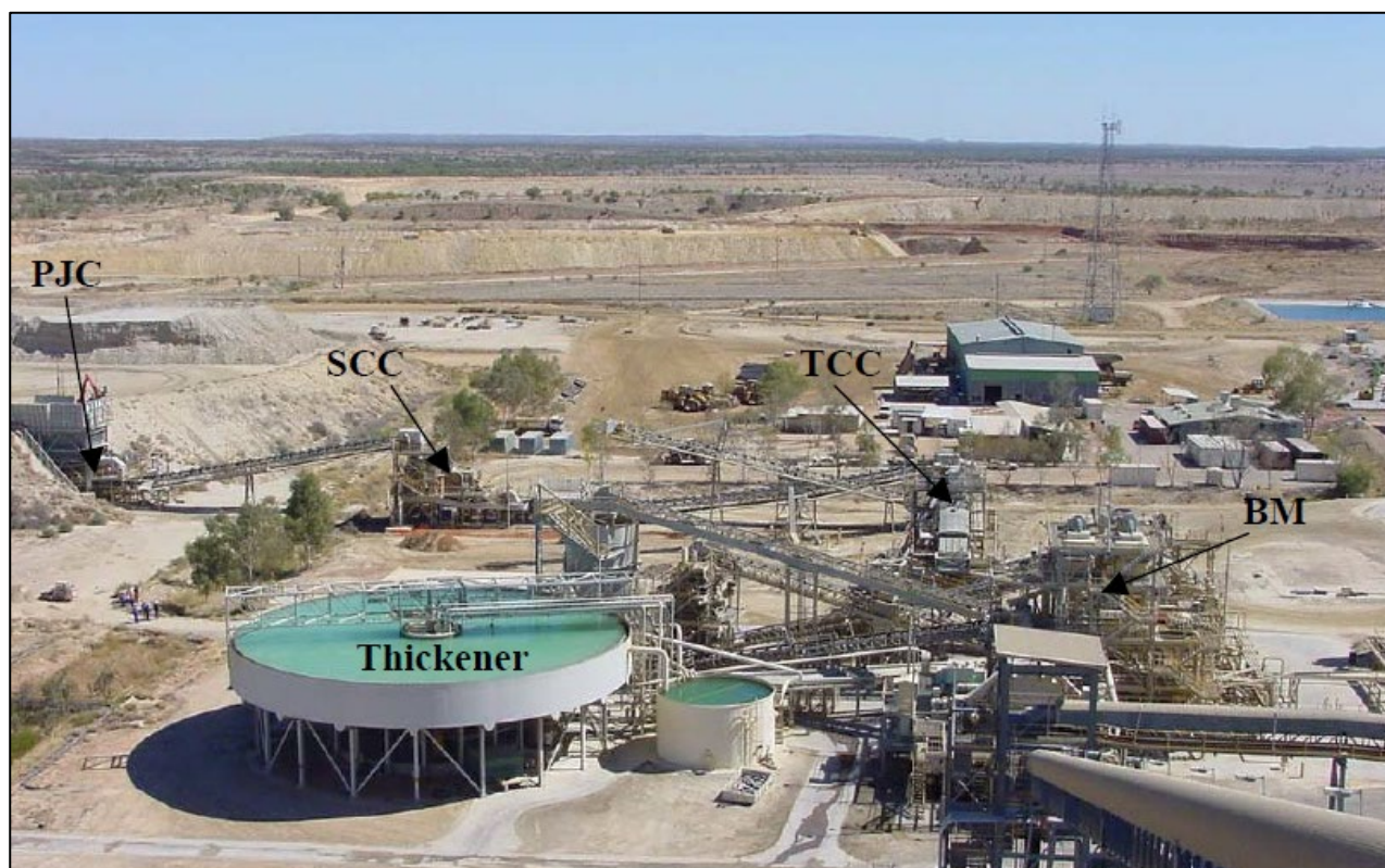
Figure 23-1. View of part of the Phosphate Hill process plant and open pit in the background, circa 2003.
