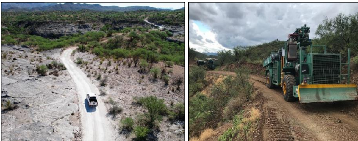
Figure 5.1 Access Road Near the Project
