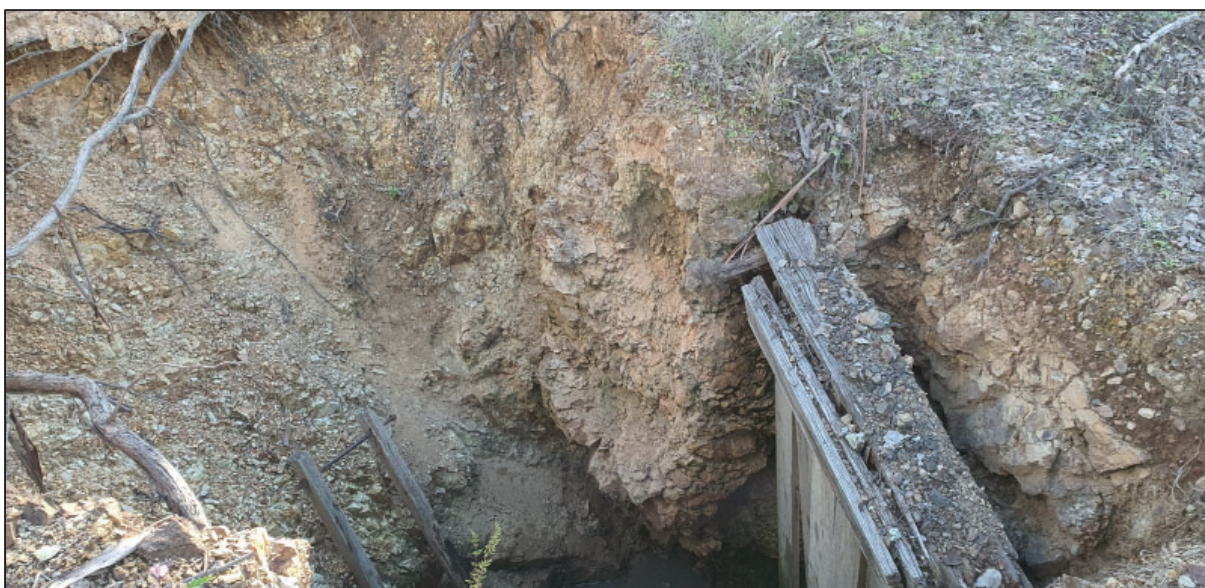
Figure O4: There are several shallow historical shafts which date back to the 1800's. They have a very small footprint are not discharging acid run-off, and are not an environmental liability.
